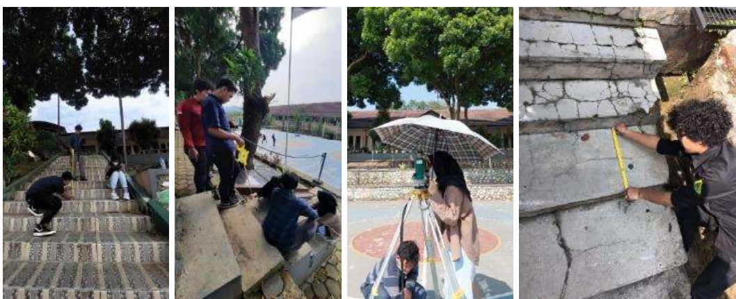
Gambar 9. Proses Pengukuran Tribun Eksisting
